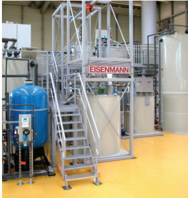
This continuous treatment plant for precipitating fluoride from waste water was pre-assembled at Eisenmann.
