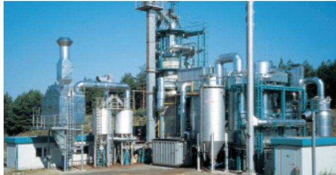
Fully automatic stationary plant with a moving bed reactor for the disposal of 30,000 metric tons of unexploded ordnance.
